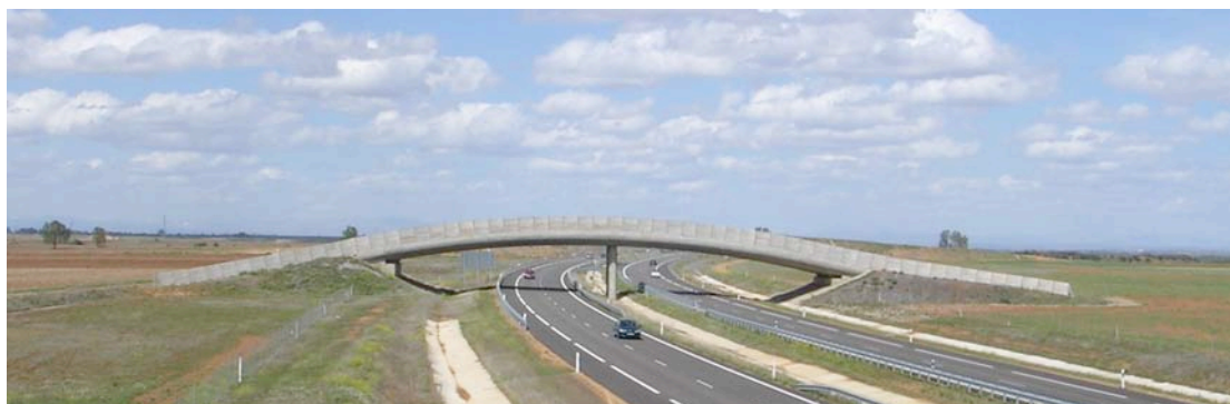
Figure 1.4. Modern fauna overpass on A66 motorway in north-west Spain (Photo: Cristina Mata)
