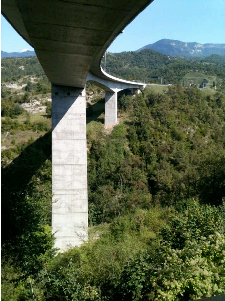
Figure 6.2. Les Salines viaduct on C37 road in northern Catalonia. This 269m long structure was designed to avoid the sensitive stream within the valley by the use of only three pillars and with construction of the carriageway being undertaken completely above the ground
