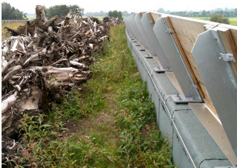
Figure 7.10. Rows of tree-roots as habitat on overpass (Netherlands)
