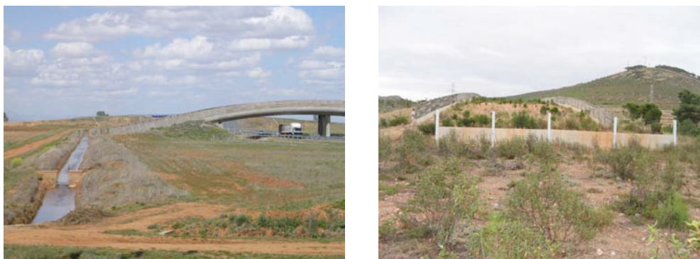
Figure 7.7. Examples of post-construction loss of connectivity caused by independent actions at the end of fauna overpasses (both from Spain). In both cases, the construction of irrigation pitches (left) and the imposition of a concrete barrier (right) resulted from poor engagement with local landholders (Photograph: Cristina Mata)
