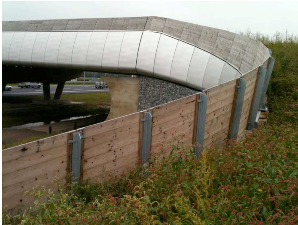
Figure 7.8. Recent sound and noise barrier structure on fauna ecoduct in The Netherlands.
