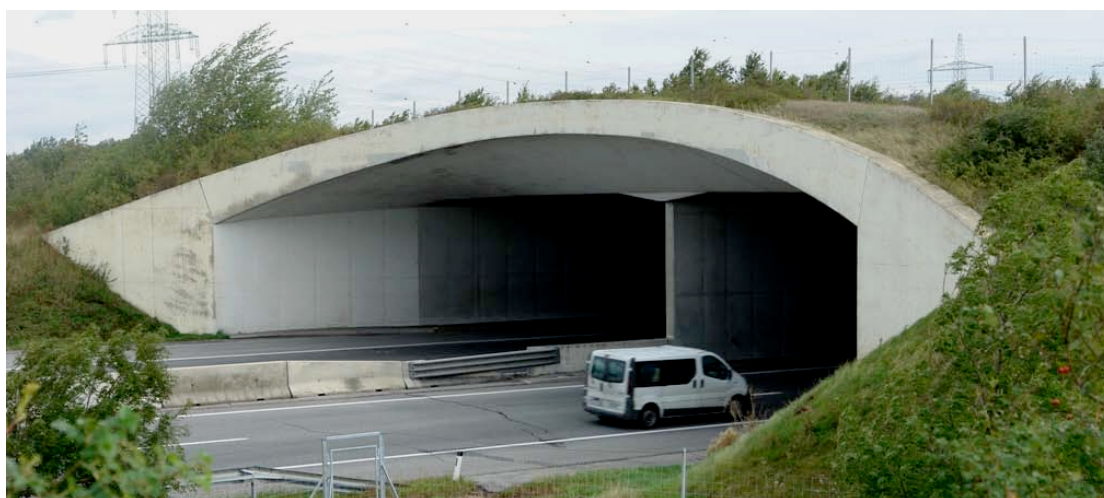
Figure 1.3. Typical open fauna ecoduct from eastern Austria (photo: Fabrice Ottburg)
