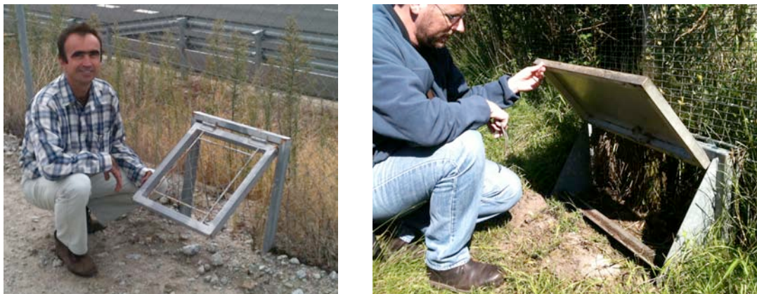
Figure 7.2. Two typical escape hatches at the base of exclusion fencing. Both require an animal on the road-side of the fence to locate the device then push with the head to open the hatch. (Left: J. Malo, near Madrid in Spain; Right: E. van der Grift, The Netherlands)
