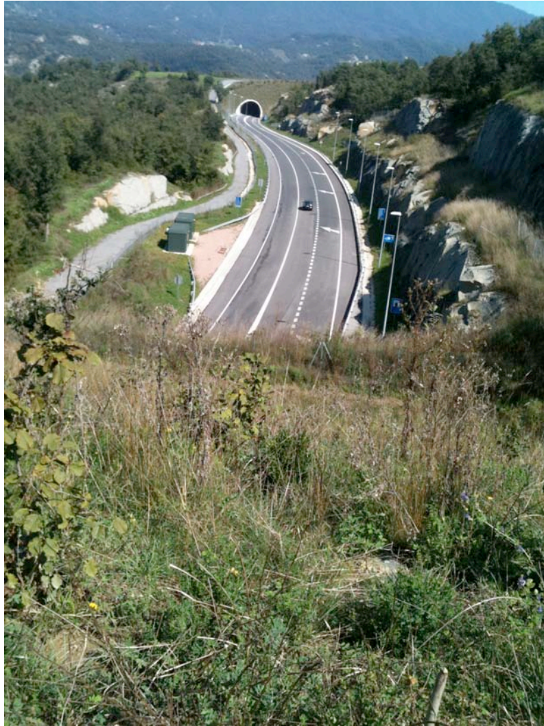
Figure 1.1. View of a section of the C37 motorway in northern Catalonia, Spain taken from the top of a 500m width 'landscape ecoduct' and looking toward another cut-and-cover style overpass. Part of Europe's most permeable road (see Box 2)
