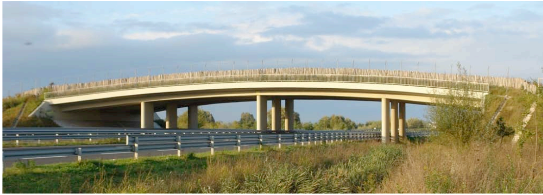
Figure 1.2. Fauna overpass designed mainly for roe deer on motorway M7 in southern Hungary
