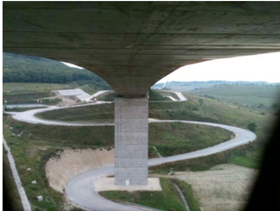
Figure 6.3. An example of an otherwise excellent viaduct in Hungary, constructed by the pillar-centric process but with all potential connectivity benefits cancelled by post-construction service roads and drainage ditches
