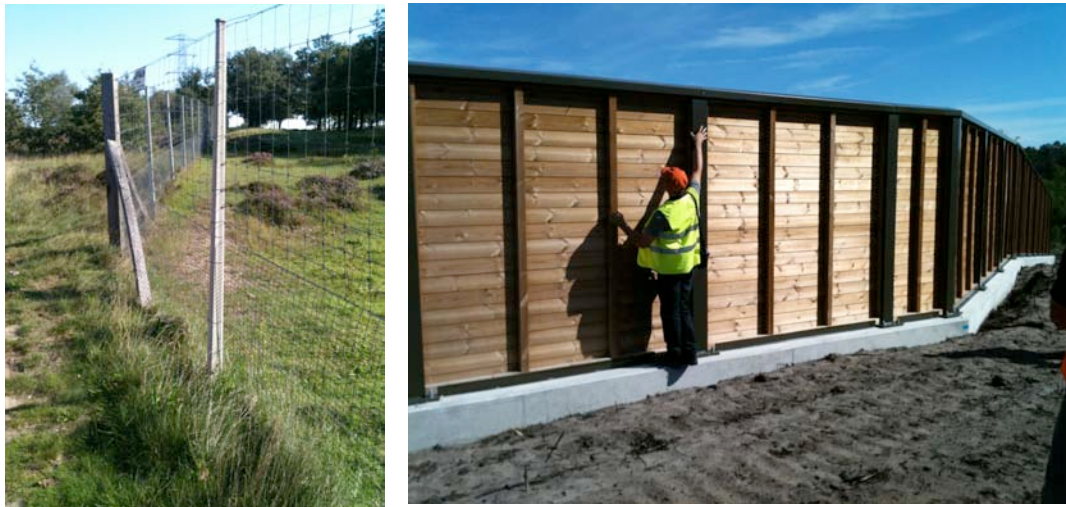
Figure 7.1. Two different approaches to fencing for roe deer. Left: Typical roe deer fencing beside motorway with lower level of mesh to exclude smaller species. This fence extended 30cm below the surface (The Netherlands). Right: Combined roe deer fence and sound and noise barrier on a game-specific overpass in southern France
